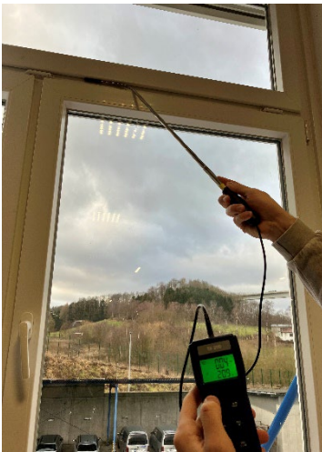
Fig. 15: Leakage detection on the window frame
