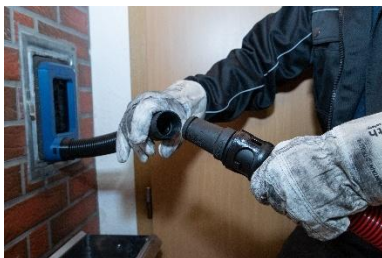
Fig.17 : Connecting the vacuum cleaner to the hose adapter
