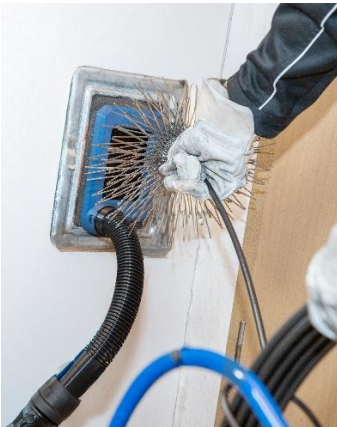
Fig.20 : Insert the cleaning tool into the exhaust system through the Wöhler SweepGate
